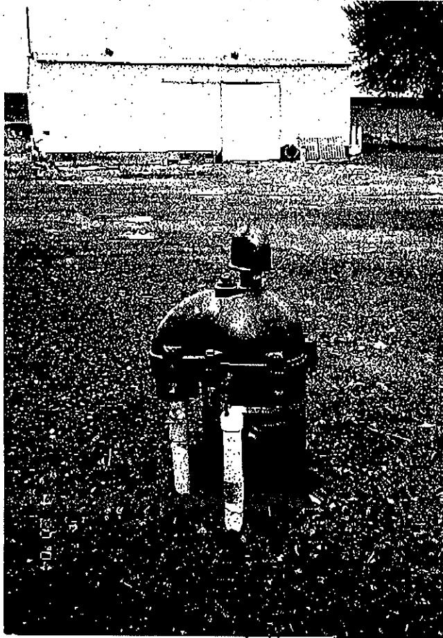
Well #9 Wellhead with Pitless Adapter Unit
