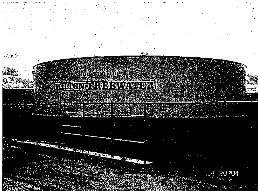
South Zone/Hwy 11 Two Million Gallon Reservoir
