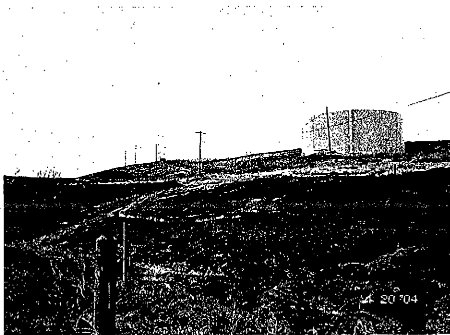
Middle Zone/SW 8 th Street One Million Gallon Reservoir
