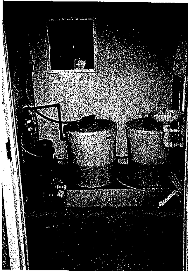
Well #9 Chlorination Room
